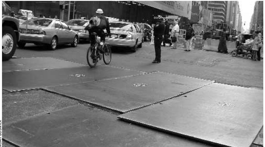
Misaligned and slick plates like these are illegal—and everywhere in NYC.
