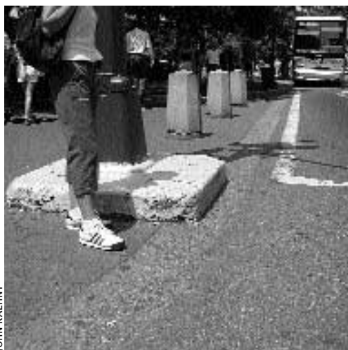
Inexpensive traffic calming at Yeshiva University in Northern Manhattan: The DOT refused to use inexpensive techniques like this to test the effects of narrowing streets and widening sidewalks.
