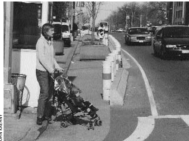
Bollards at 59th Street and 5th Avenue in Manhattan: Bollards are an attractive and inexpensive way to enlarge pedestrian space without expensive drainage work. The DOT refused to consider designs like this in its Downtown Brooklyn traffic calming study.
