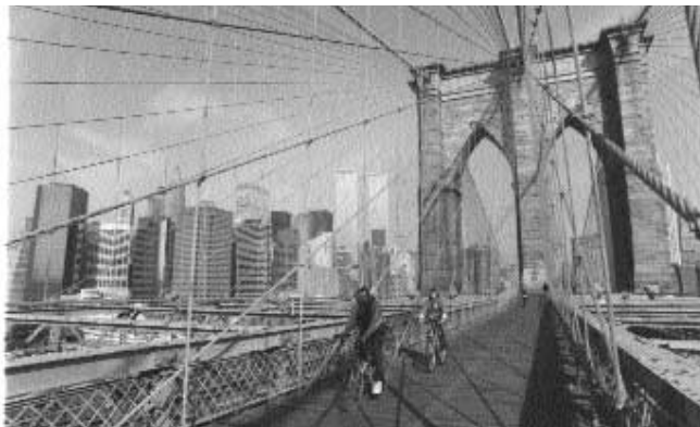
The barely visible Brooklyn Bridge lane divider needs repainting.
