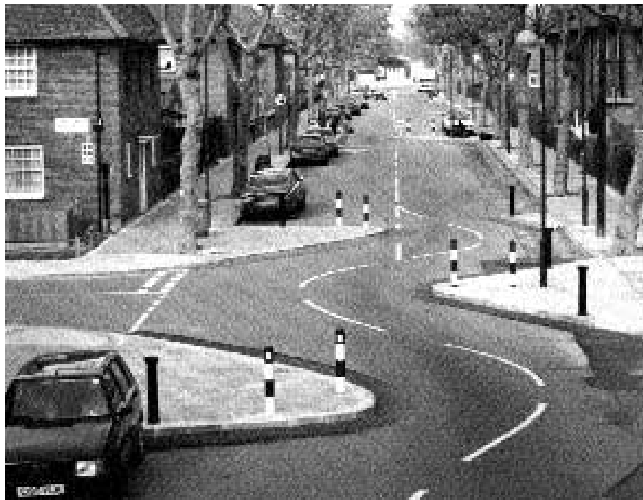
This busy residential street in Sheperds Bush had a high accident rate and too many speeding cars. Here, chicanes, and pinch points, stand out to force slower speeds.
