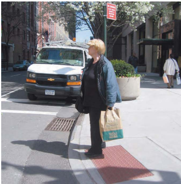
Upper West Side: New ADA compliant curb-cuts
