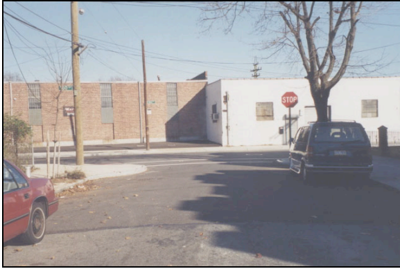
Figure 3: Curb Extension to Discourage Turning Trucks, 180 St, Queens
