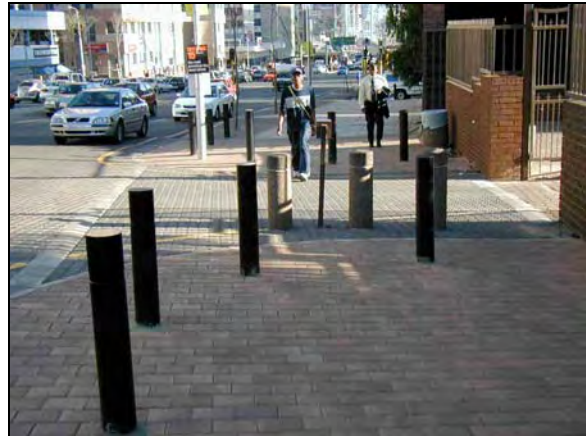
Figure 13: Bollards Along a Driveway
