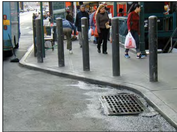
Figure 15: Bollards Protecting Subway Entrance, Manhattan
