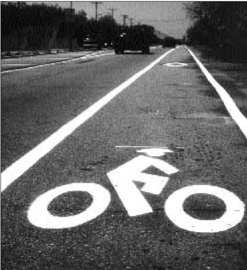
New bike lane on Rockaway Point Boulevard serves as traffic calming by narrowing street from four lanes to two. DOT also installed rumble strips.
