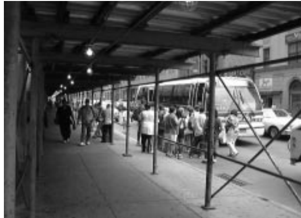
Scaffolding at 370 Jay Street.
